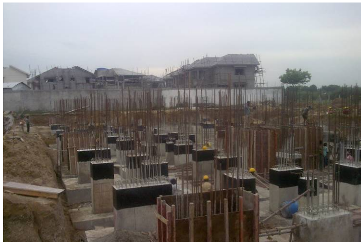
Site work under progress
