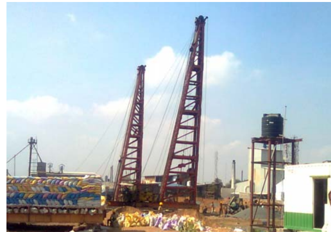
Work under progress
