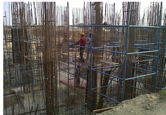
Work has reached Ground Level
