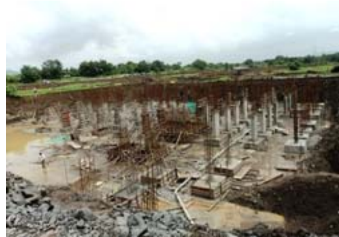
Basement work under progress
