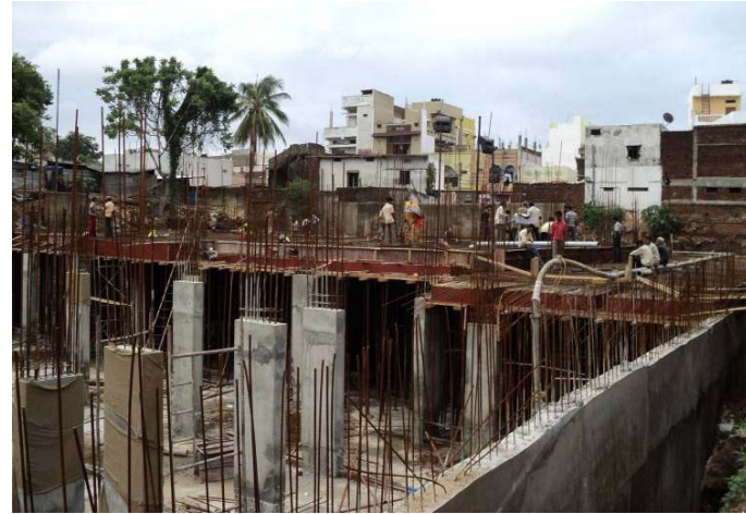
Basement work under progress
