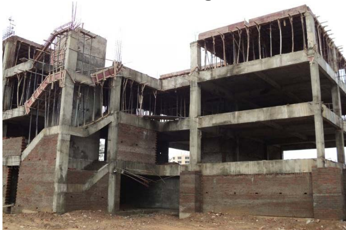
Work under progress
